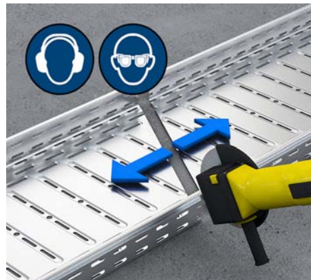
11 | Horizontal change in direction For a horizontal change in direction without normed formed components, mitre the cable tray as required, deburr and cold-galvanise it.
