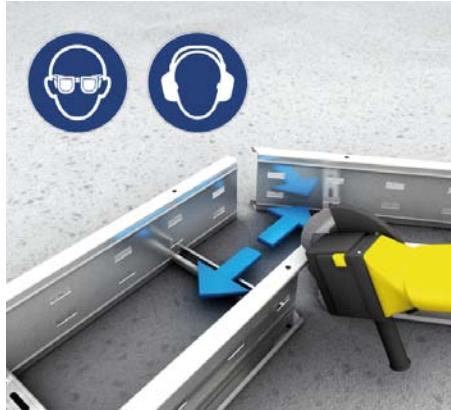
17 | Horizontal directional changes For horizontal directional changes of more than 30° note, that you have to create a mitre joint for the wide-span cable ladder at the required angle, then, as necessary, remove any extra rungs. Afterwards deburr and cold-galvanise.
