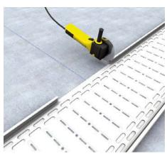
**4** | **Junction** In order to create a junction, notch the duct bottom piece according to the width of the duct branch.
