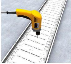
**3 | Fixing** Mount duct to the rough concrete in one place per length using plugs.
