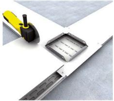
11 | Dummy covers Cut dummy covers UKD accurate to measurement, place on the duct and then latch in.
