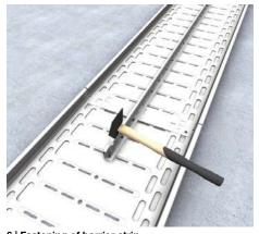
**6 | Fastening of barrier strip** Barrier strips must be mounted in parallel offset of the duct.
