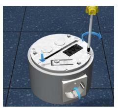
**7 | Assembly after light-current installation**After the complete installation, screw the floor plate or, if so, the cover plate with the tube outlet.
