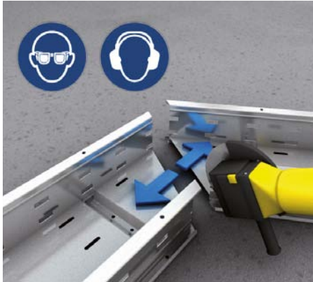
16 | Horizontal directional change Horizontal turnaround > 30 degrees – closed tray bottom. Mitre wide-span cable tray as required, deflash and
